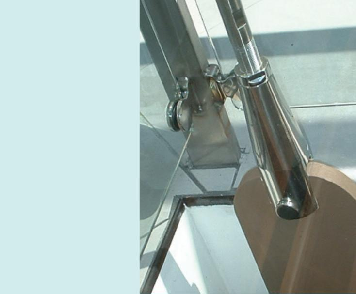
SBS-450 forks and pins are manufactured from Duplex grade stainless steel. This offers high resistance to corrosion and superior mechanical properties over marine grade 316 (EN10088 1.4401).
