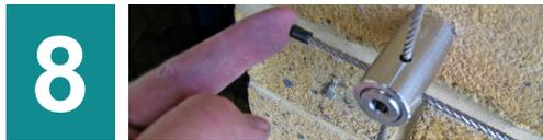
8 When you have finished tightening all the hubs the cable ends can be cut to size. Then attach the plastic cable caps to the bare cable ends on the outside edges
