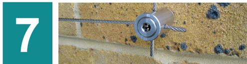
7 Once all the wires are in place and hand tight, you can then start to tighten with the allen key, work from the outside edges, sequentially, into the middle. When you are tightening the central screws the cable is pushed into the barrel of the hub thus creating the cable tension between the hubs.
