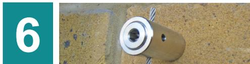
6 Start with the horizontal wires and pass them through the hubs, these will remain in place without any tightening. Once these are in place, begin to insert your vertical cables working from an outside edge of the lattice, as you pass through each hub hand tighten the central screw. Leave about an inch or so protruding from the outside edges.
