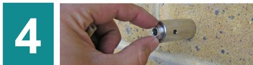
4 Secure your hubs to the wall ensuring the holes are in alignment with each other. Once all hubs are secure insert the central tightening screw loosely, so you can start to run your cable through.
