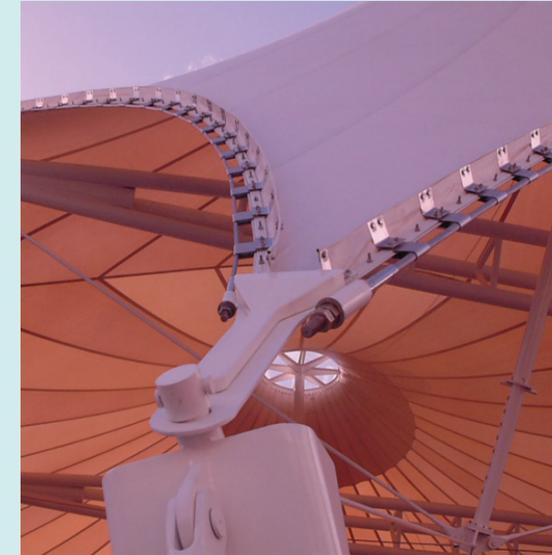
The SBS-450 tie bar system consists of a bar with a left hand and right hand threaded fork at each end.
